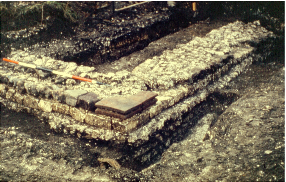
Foundations of the corner of a substantial building found at The Tene in 1968
